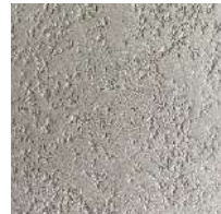
Stucco Walls Surfaces
