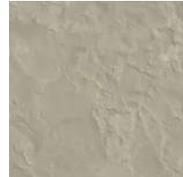
Textured Plaster Application Wall Surfaces
