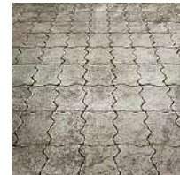
Concrete Pavement Stones Flooring
