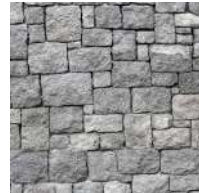
Dry stacked stone wall Wall surfaces
