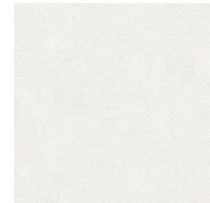
Plaster Wall Surfaces
