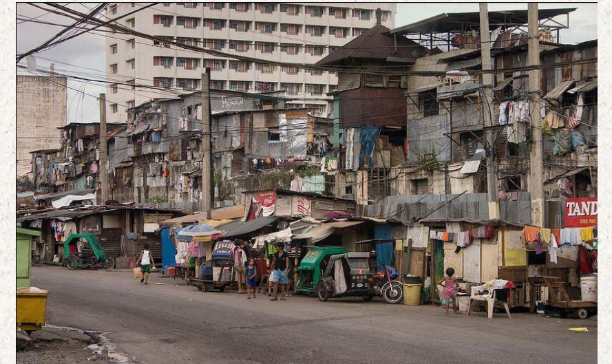
NEIGHBORHOODS IN MANILA [Anton Zelenov, Manila, Philippines, 2008, https://www.dreamstime.com/royalty-free-stock-photo-poor-people-living-destroyed-buildings-near-road-mani-mani-philippines-december-slums-illegal-settlements-image35783775 ]
