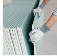
Drywall Wall Surfaces
