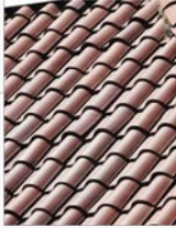
Concrete Roof Ceiling surface
