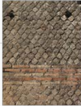
Brick Panels Wall Surface
