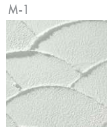
M-1 Textured Stucco Wall surface
