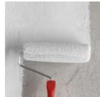
Paint and Primer Wall Surfaces
