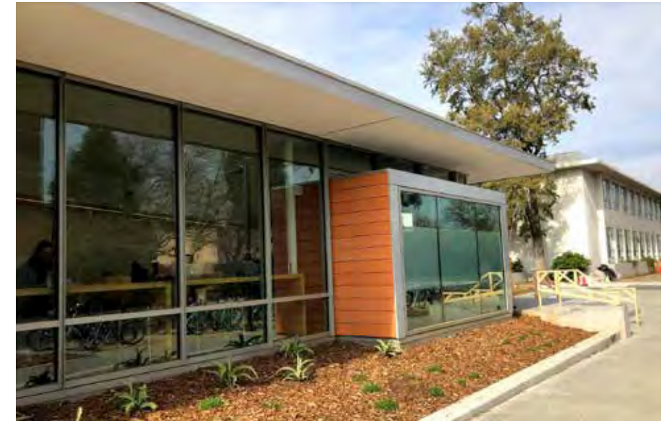
Right side features wall of glass windows and extended space.
