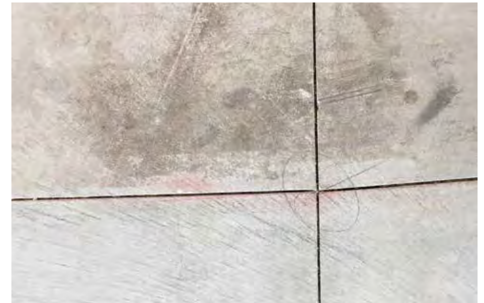
Interior — concrete floor.
