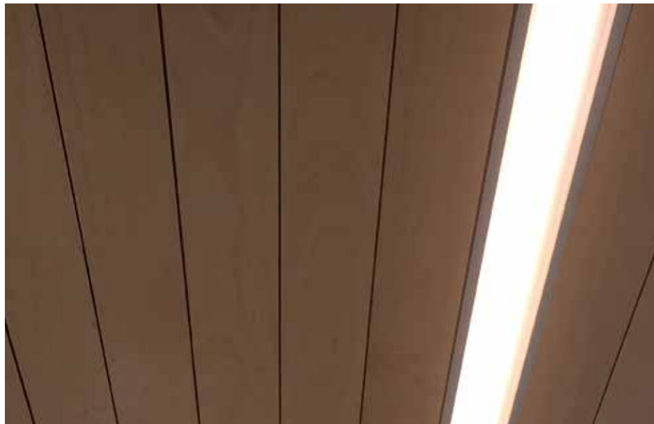
Interior — wooden ceiling panels.
