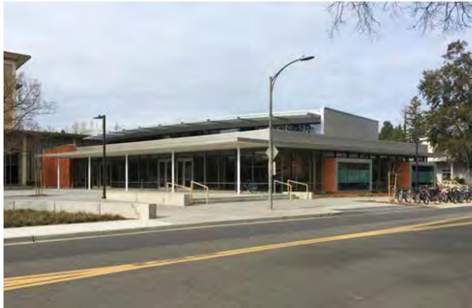
View of building from across the street.
