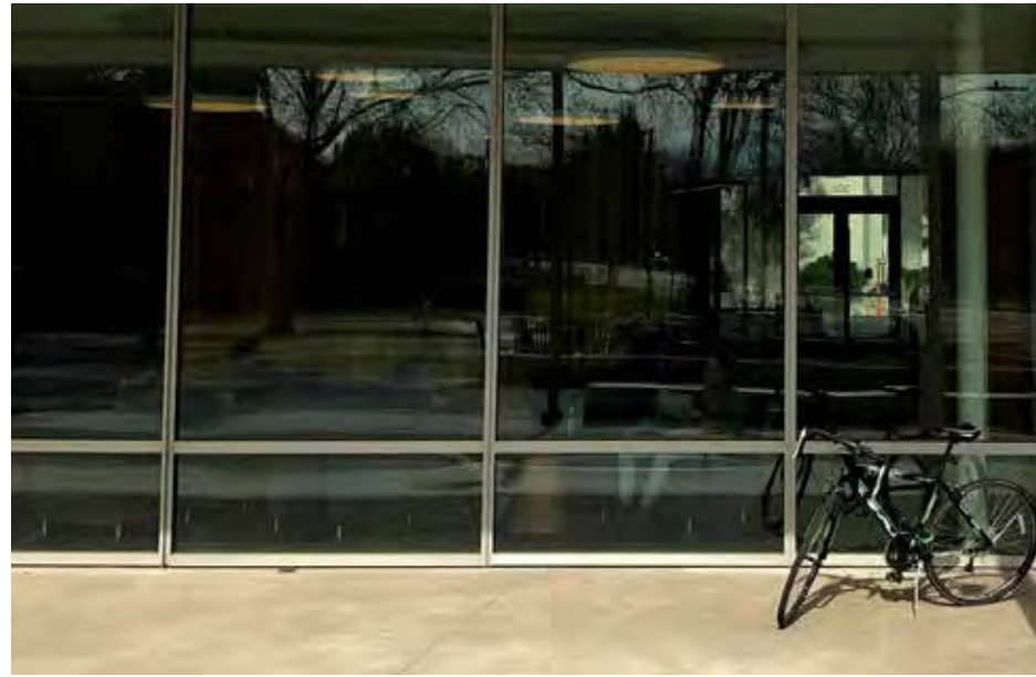
Exterior — glass windows and concrete floors.
