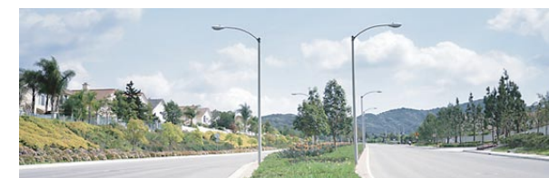
39 Weir Canyon Road, Street Lighting March 2004, City of Anaheim, CA
